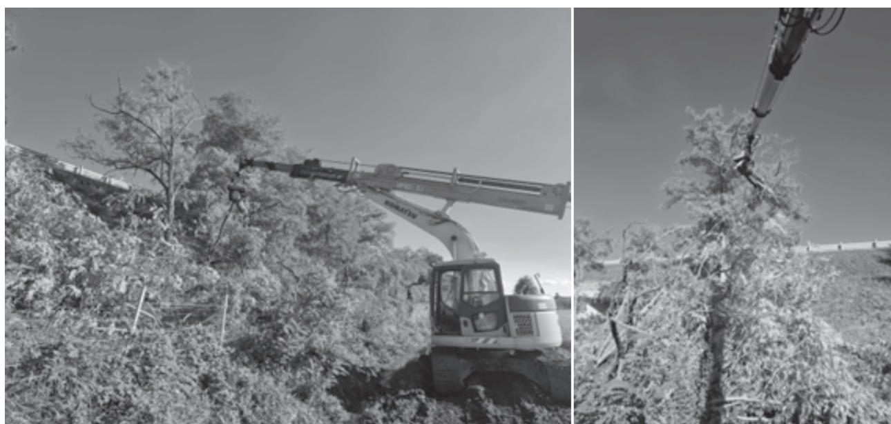
Fig. 5 Specific machine at work in highway embankment
