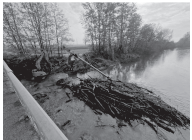
Fig. 10 Removal of logs near a bridge
