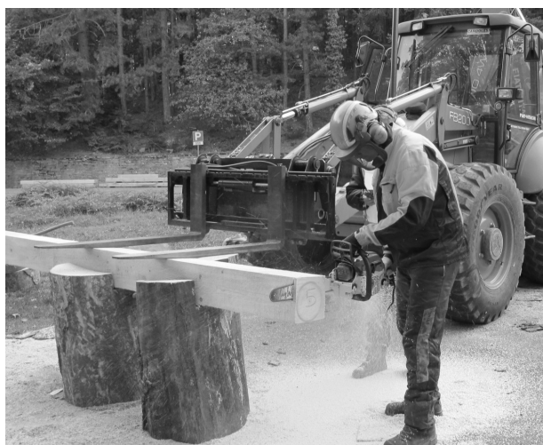
Fig. 4 Tractor holds a wood beam on wood supports while the operator performs cross cutting
